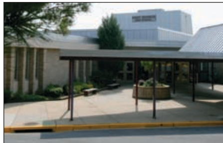
Paint Branch HS
