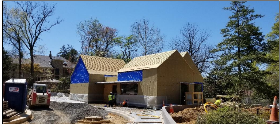
The Josiah Henson Park Visitor Center/Museum is under construction.
