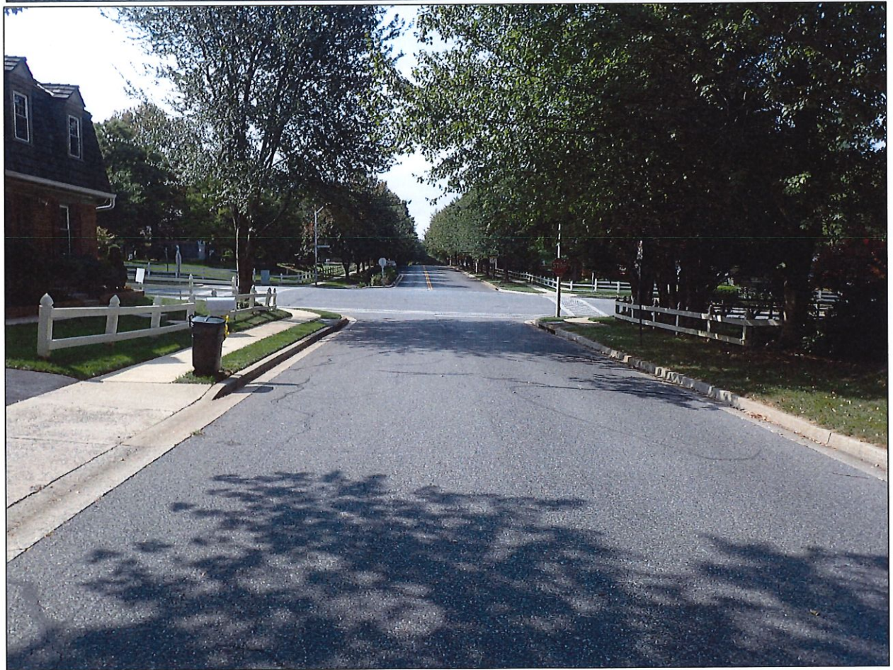
EB Bristol Downs Dr approaching Saybrooke Oaks Blvd
