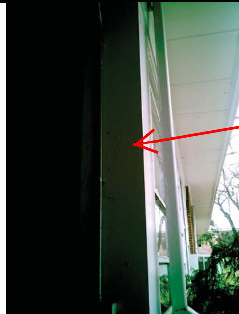
Picture 8: White Metal Wall Casing
