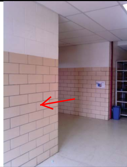
Picture 6: Tan CMU Wall
