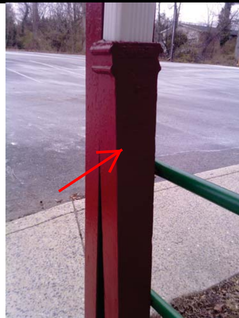
Picture 12: Red Metal Gutter Pipe
