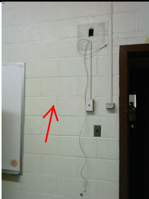
Picture 3: White CMU Wall
