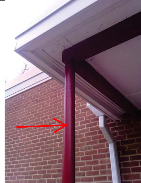
Picture 14: Red Metal Column
