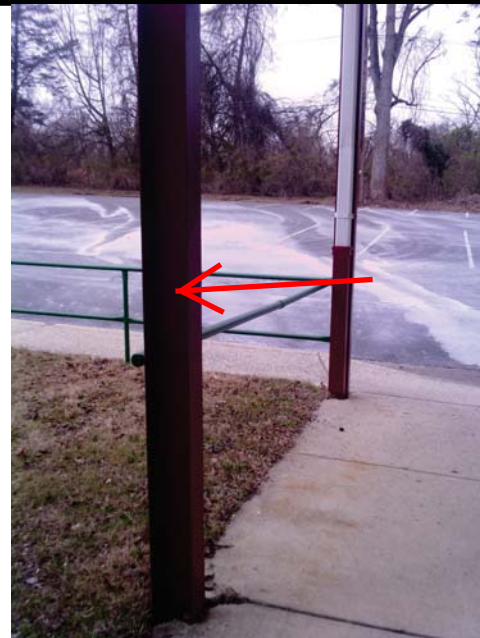
Picture 10: Red Metal Column
