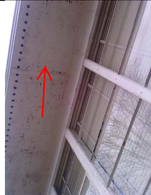
Picture 16: White Wood Soffit
