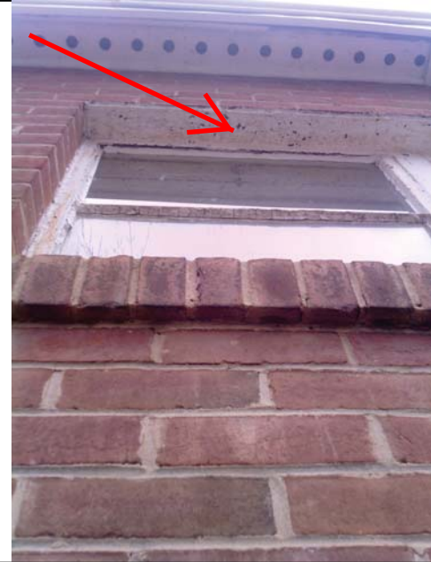
Picture 18: White Metal Window Lintel
