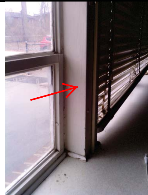
Picture 4: White Metal Window Casing
