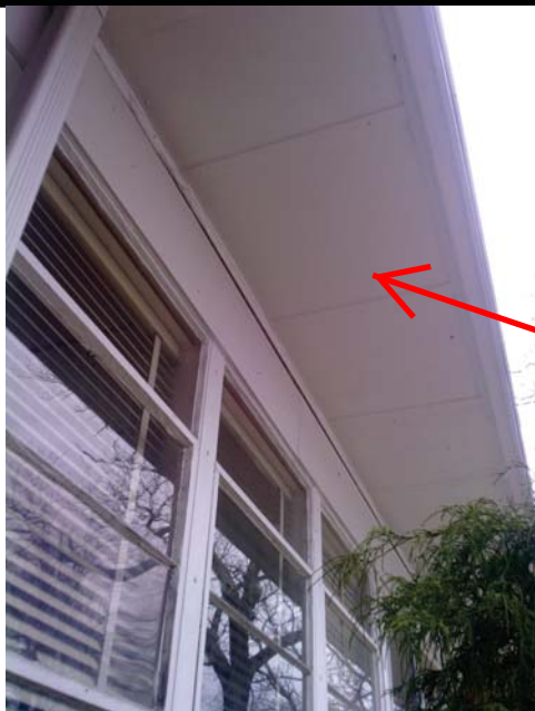
Picture 11: White Wood Soffit
