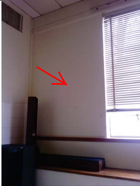
Picture 1: White CMU Wall
