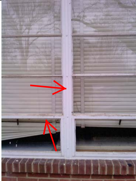
Picture 13: White Metal Window Casing
